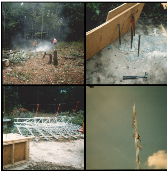
Tower Reconstruction after damage created challenges along the way.
